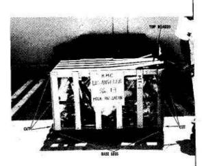
Pull down the two ends of the crate, and then pull down and remove the two sides. Lift the front end of one unit, and then roll it out of the crate base. CAUTION: Peen over any crate nails which could puncture the tire.
